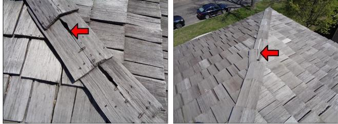
Apparent hail damage was noted. We recommend review by the appropriate insurance carriers and repair by a qualified roofer to the extent necessary to assure that the roof is both serviceable and insurable.
